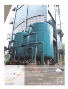
The water from the open well is pumped to a water chlorination tank from where it is chlorinated and pumped to an overhead tank. It is distributed from here to all the institutions in the campus.
